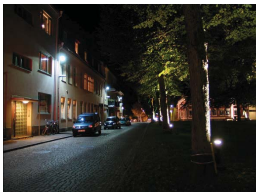
Figure 1. Street light at 6 metres height.
