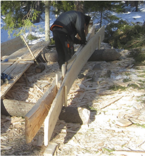
Figure 5. Production of roof boards. K.M. Melin.
