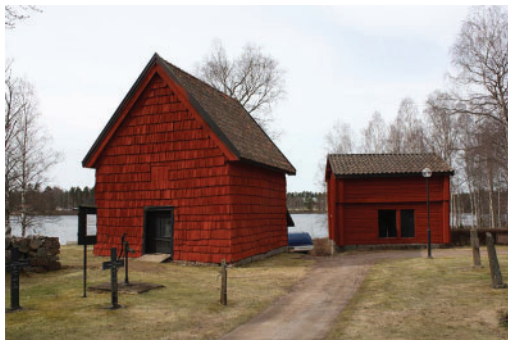
Figure 1. Ingatorp tithe barn to the left. It's plausible that the barn was built in the early 13th century for storage of tax-in-kind to support the vicarage. The crafted architecture connects to the contemporary wooden gothic churches, with boxed timber, high pitched roofs and leaning gables. The building had originally visible tarred logs and the roof was covered with tarred wooden roof shingles. In the late 16th century the exterior walls were covered with shingles as well. The building has been in active use as storage in almost 800 years. Photo: G. Almevik.
