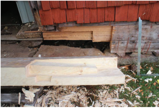
Figure 4. Surgical repair of the damaged front sill. Photo. K.M. Melin.
