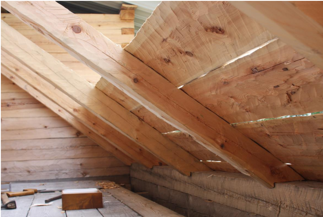
Fig. 24. The sacristy. The boards are put on the roof of the sacristy in June 2013. Compare with Fig. 8. Photo Karl-Magnus Melin.
