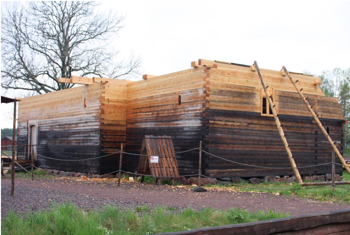
Fig. 25. The reconstruction in 2013. The nave and chancel timbered to the level of the sacristy, where the cleaved boards are placed. Photo Karl-Magnus Melin.
