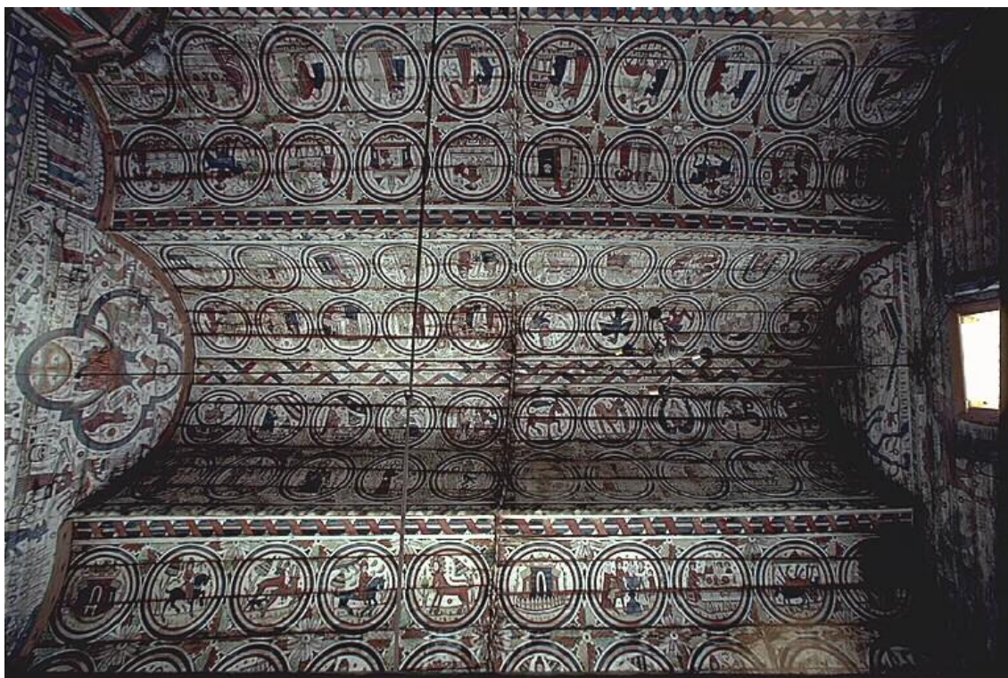
Fig. 7. The trefoil of the nave at Södra Råda. In the middle of the nave, the boards are jointed and this seam is hidden by a carved rope moulding. We have examined photos of the boards in the Södra Råda church, and all of the boards are approximately 6 metres long. Photo National Heritage Board, ATA.
